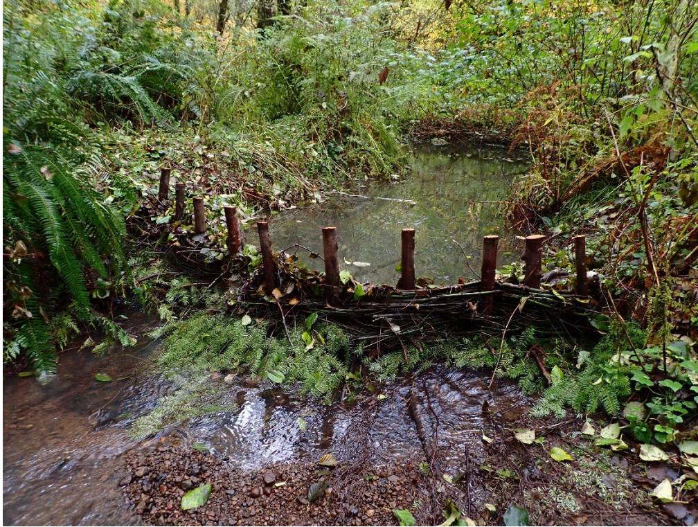
A recently installed Beaver Dam Analog in a creek in Thurston County, WA slowing down water and capturing sediment. Photo by Daniel Trovillion, WDFW.
