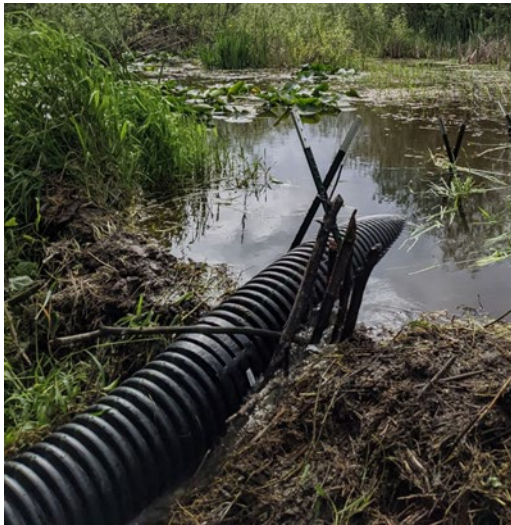
Two examples of water level control devices that have been installed through beaver dams. The photo on the right showcases how wire cages can be used to protect the pipe inlet from being plugged up by beavers. Photos by Beavers Northwest.
