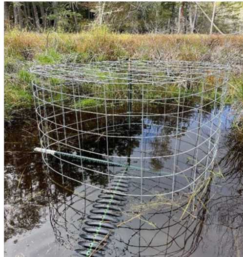
Two examples of water level control devices that have been installed through beaver dams. The photo on the right showcases how wire cages can be used to protect the pipe inlet from being plugged up by beavers. Photos by Beavers Northwest.
