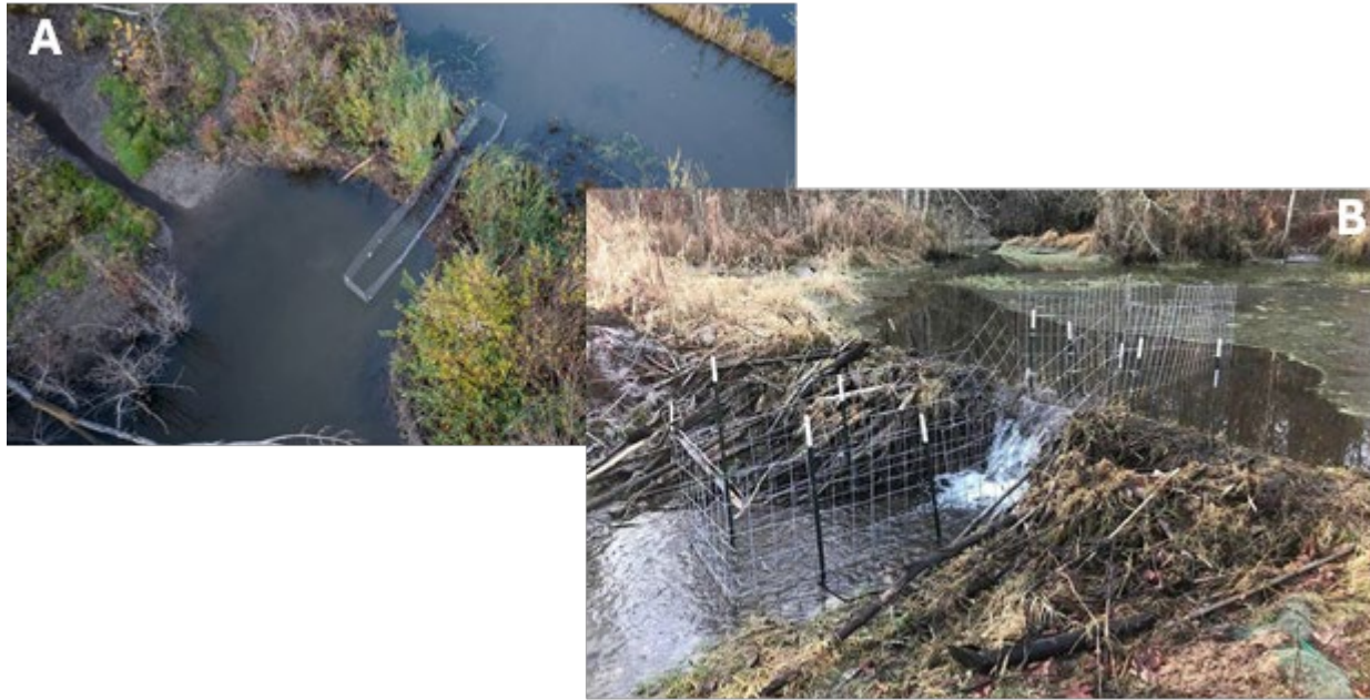
(A) Aerial view of a notch exclusion fence through a beaver dam. Photo by Kenny Katz and (B) ground view of a notch exclusion fence through a beaver dam. Photo by Beavers Northwest.
